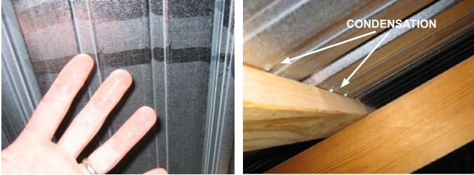
Photos above show the heavy attic condensation that can be caused by opening attic access panels. Warm and moist bird air condensing on roofing panels, as in left photo, will lead to premature rusting. Drips onto lumber, as in the photo of the purlin at right, lead to premature rotting of the roof support structure. Condensation can also cause major damage to insulation. Opening attic panels is not likely to melt enough snow off the roof to be worth taking the risk of major condensation damage.
