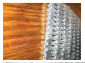
This is a close-up photo of a roof truss gang nailing plate. Notice the metal plate separating from the lumber truss member, especially at the top of this picture. If the house is put under a heavy snow load, this loosened truss plate coud lead to failure of the truss, which in turn could cause the entire roof to fail. Routine inspection of truss plates for damage or loosening, and prompt repairs if such problems are found, is essential to avoid potential snow disaster.
